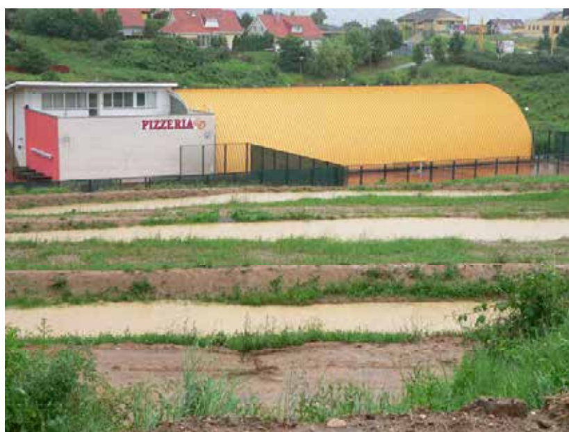
Fig. 36 The KVP housing estate in Košice – protection of buildings under a slope with the help of earthen bunds along contour lines
