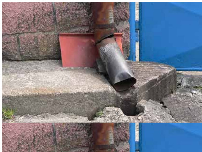
Fig. 13 The sluicing away rainwater
